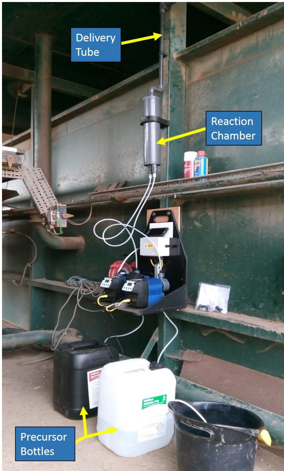
Figure 13 Automated chlorine dioxide delivery system installed on farm. Visible are two precursor ingredient bottles pumped into a grey reaction chamber from where the chlorine dioxide gas flows to the hot water tank.
